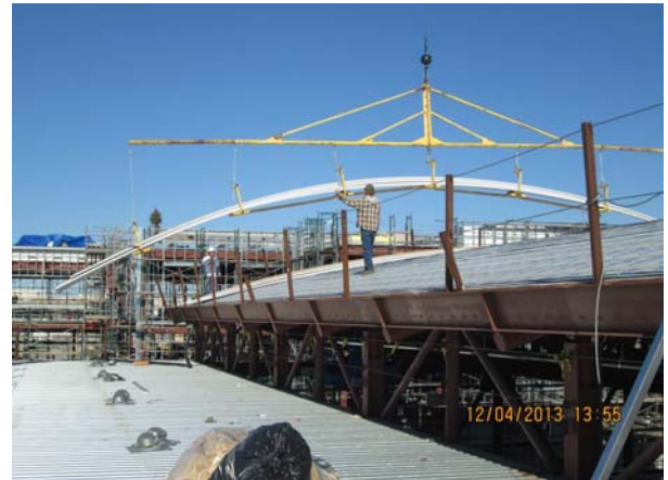
Building B - Roofing
