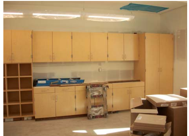
Building B - Casework Installation
