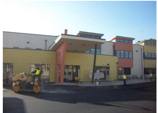
Front of Building A w/AC Paving
