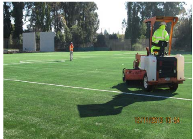
Futsal Field installation
