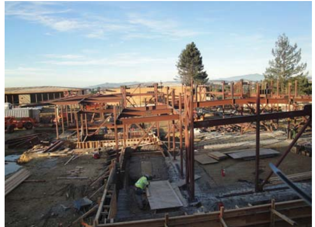
Building D Structural Steel
