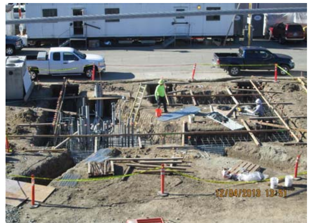
Site Work - Utility Yard Foundation
