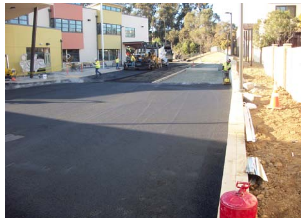
AC Paving in front of Building A
