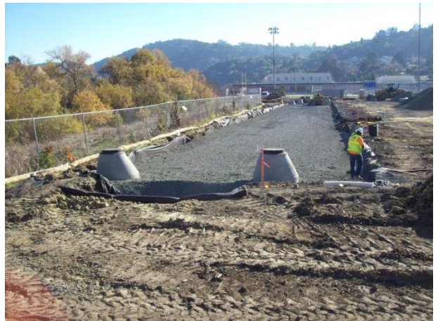
Installation Of Manholes
