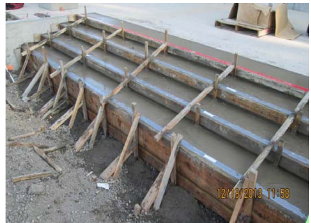
Concrete Stairs between the school and the Futsal field
