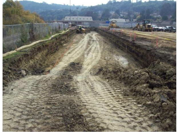
Excavation for Detention Basin
