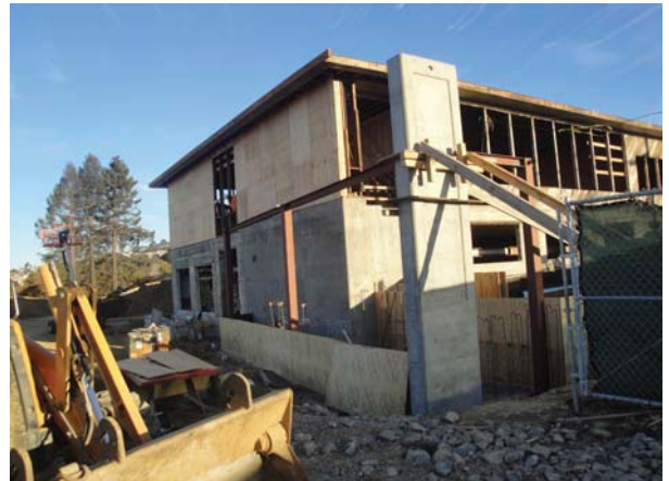
Building A Exterior Shear Wall
