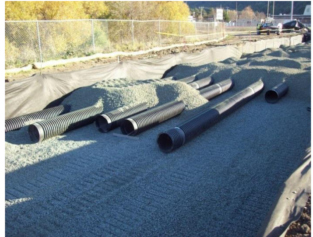
Installation of Pipe In Detention Basin
