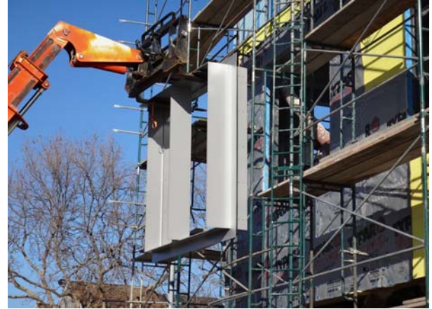
Building A - Shadow Box mock-up installation
